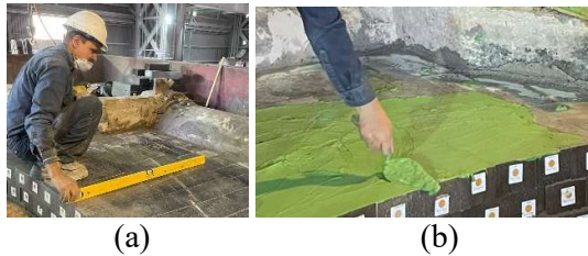
Fig. 3 (a) check the flatness, (b) mortar patching.
