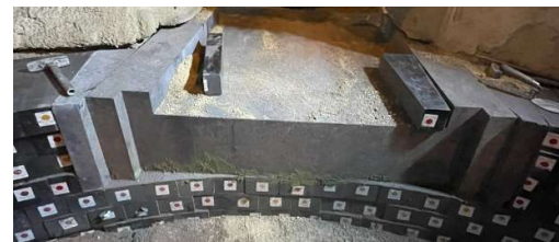
Fig. 6. Prefab slag door solution after mounting the upper shell.
